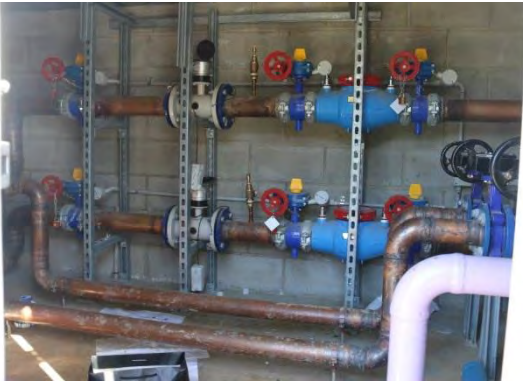
Figure 2: Hydrant Booster Plant
